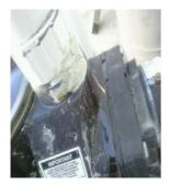
**Location:** Exterior Right **System:** Exterior **Condition:** Pool equipment leaks.
